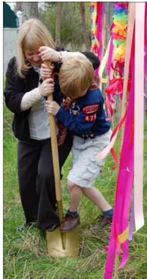
(Left) Cara Leckenby and son Calvin teamed up to break ground on 21st Street at the April 27th groundbreaking ceremony for HFHEJC’s 16th house
