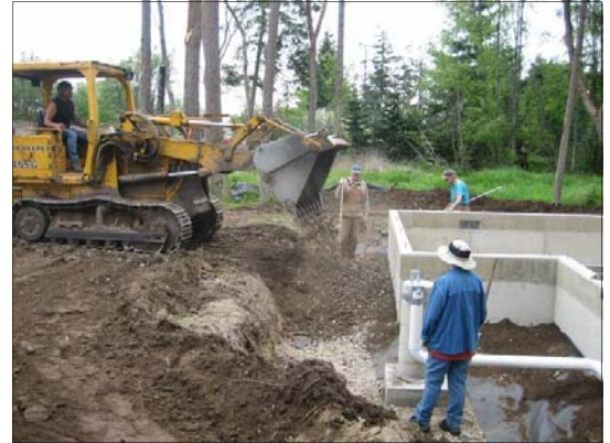
Subcontractors and volunteers work together to backfill the Leckenby foundation
